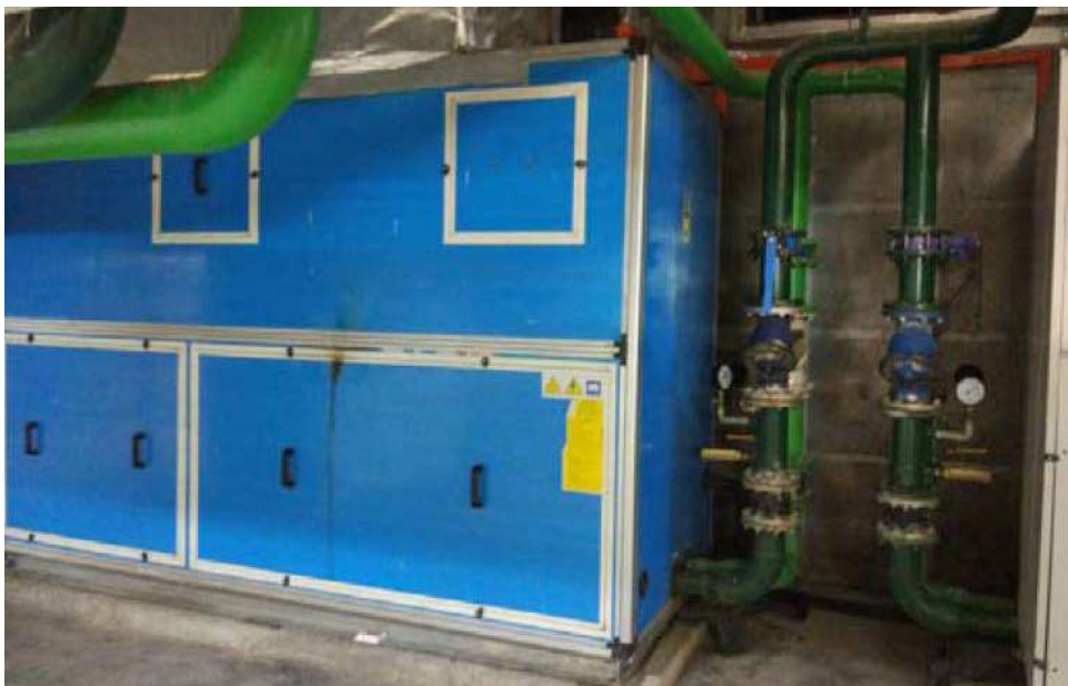
Figure 5: A Water Cooled Packed Unit (WCPU) in AHU room.
